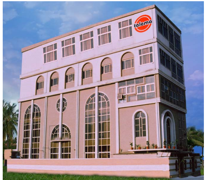
Talema Electronic (India) - Chokes & Inductors - Production Hall
